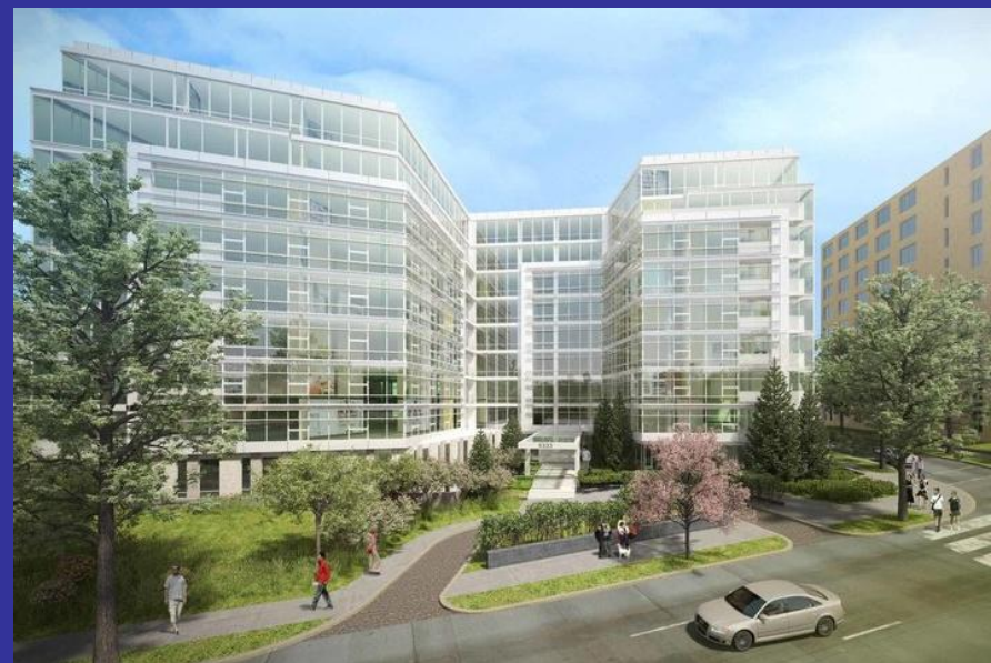
Under construction: 5333 Connecticut Ave. NW in affluent Chevy Chase by Cafritz. 19 IZ units: 10 at 50% AMI, 9 at 80% AMI, Source: http://5333connave.com/
